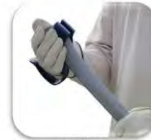
Figure 14. Slider tool being used to facilitate installation
