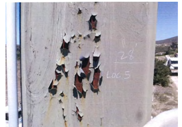
Damaged Coating
