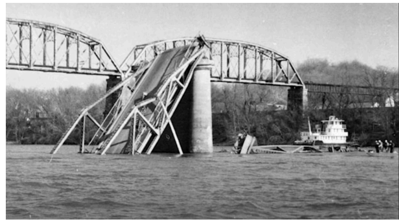
Silver Bridge Failure
