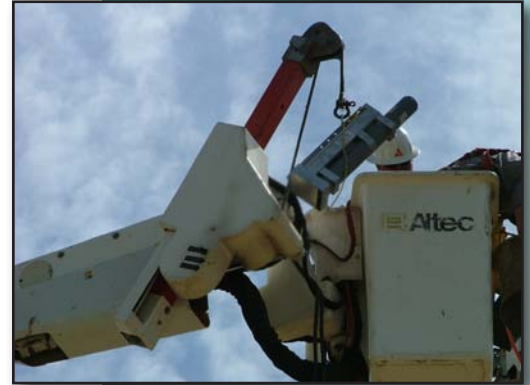
Georgia Power transmission construction lineman making conductor sleeve.
