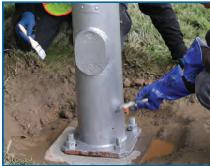
Application of corrosion-resistant coating
