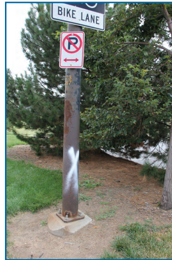
Corroded pole
