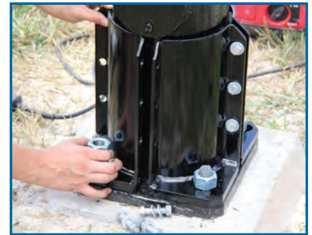
Installation of repair sleeve
